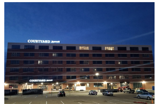
Courtyard Marriott Waterloo Cedar Falls
